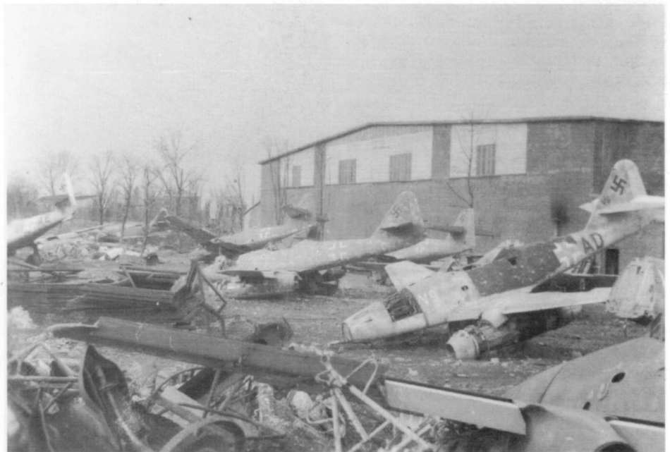
The sad fate awaiting the majority of the more than 1,400 Me 262s produced by the Messerschmitt Augsburg and Regensburg factories as time runs out for the Third Reich. The simplest way to disable the jet was to smash the forward landing gear leg. Aircraft in the foreground is the high speed prototype V9 (V1 + AD) completed in January 1944 and used for communications testing.
